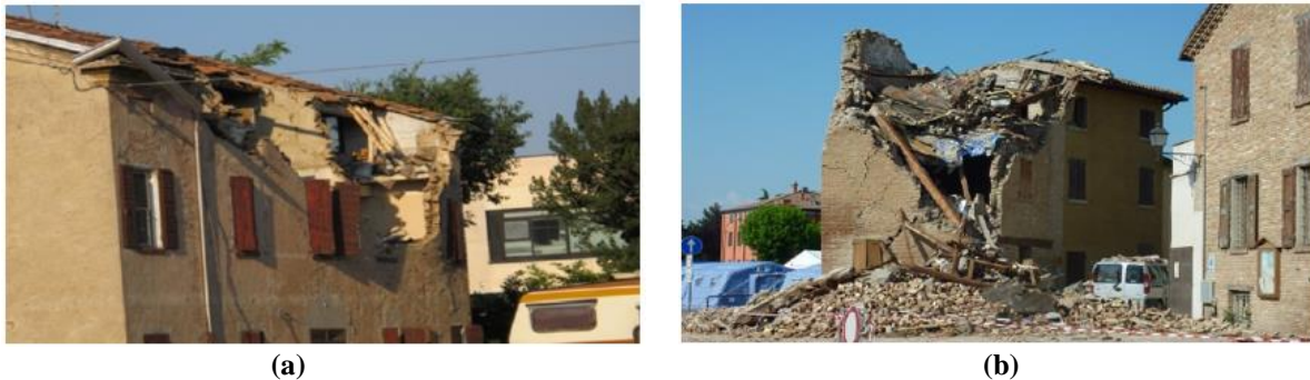
Fig. 1: (a) 2012 Emilia earthquake: collapse due to the absence of connections between floor/diaphragm and masonry walls; (b) collapsed due to the absence of efficient floor and roof diaphragms
